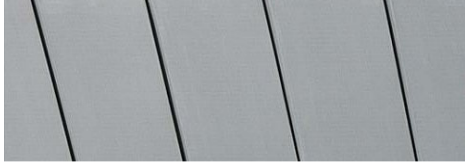
Zinc clad (non-combustible) external bathroom addition to match existing kitchen pop-out
