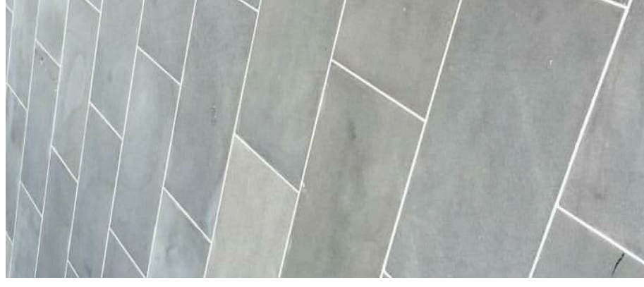
Large format stone paving to terrace
